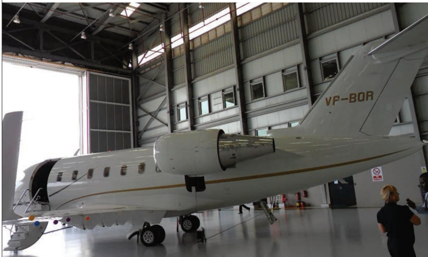
Saving millions of dollars: Aero Contractors' MRO facility, at Murtala Muhammed International Airport in Nigeria, became operational in 2018 and has carried out heavy maintenance for various airlines.
