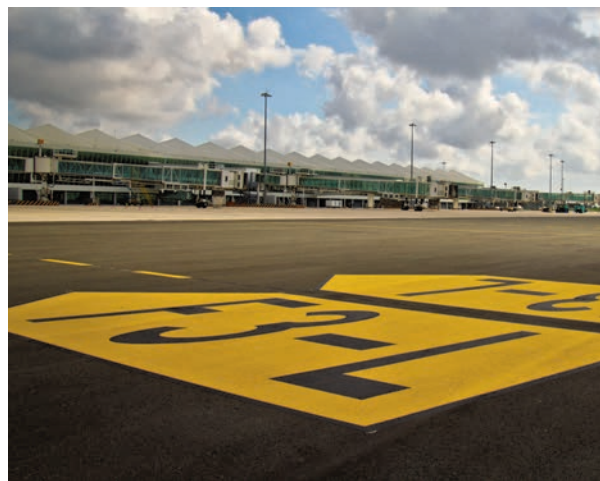
Bridging the gap: The new terminal has eight airbridges to help speed passenger flows on and off aircraft.
