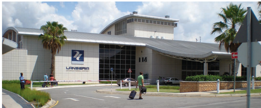
The airport handles over two million passengers annually.
