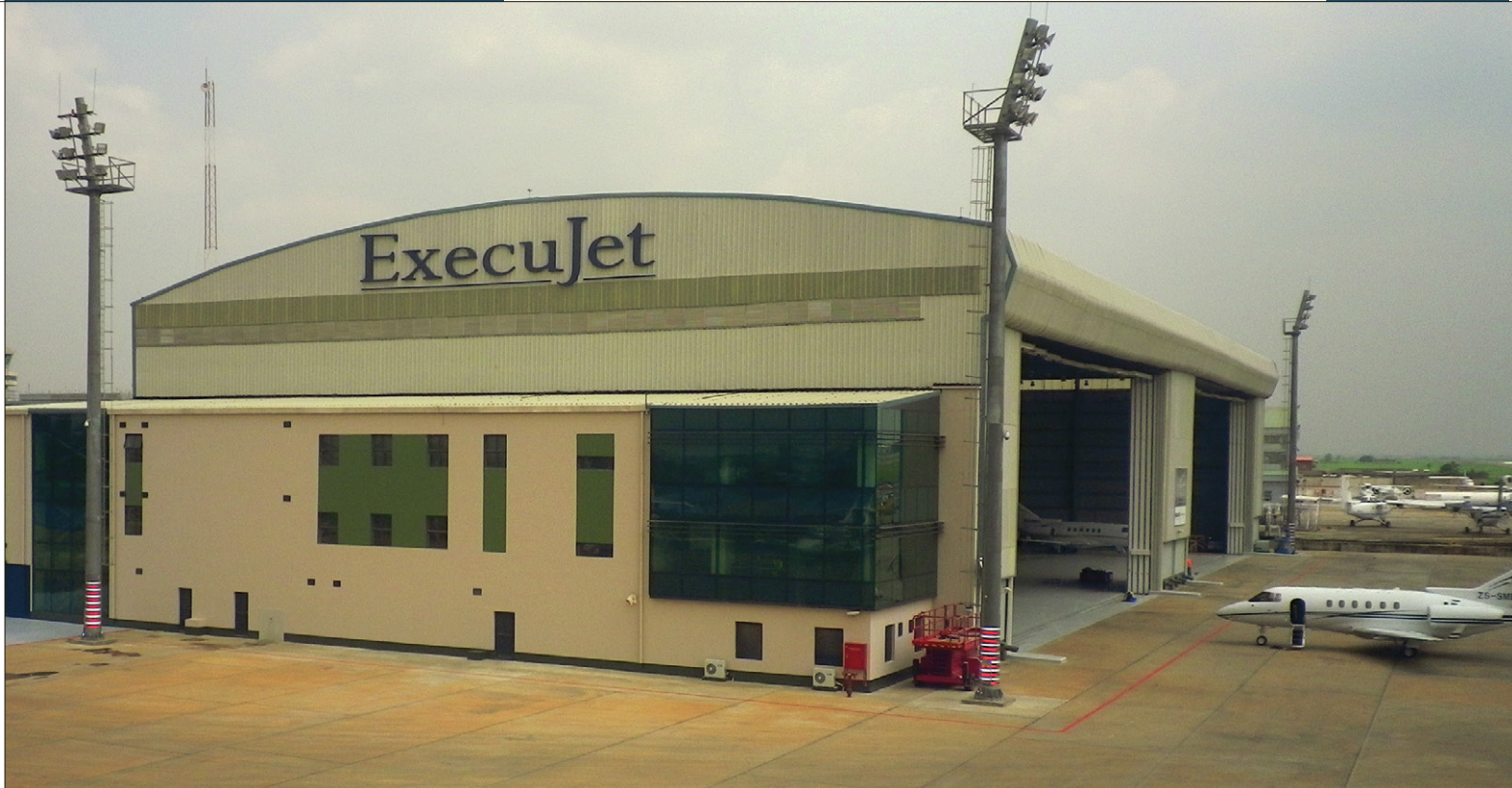
ExecuJet Aviation Group is adding a Falcon 900B, Hawker 800 and Bombardier Challenger 604 to its managed fleet. Pictured is the company's relatively new Lagos facility.
