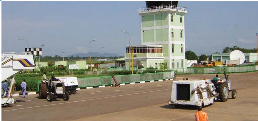
South Sudan signed a $158 million contract to upgrade Juba International Airport but progress is slow.
