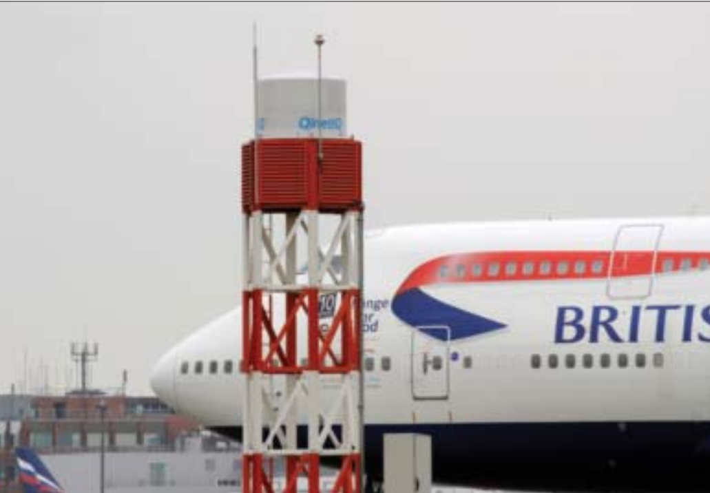
DXB has been fitted with the state-of-the-art QinetiQ FOD detection system- Tarsier.
