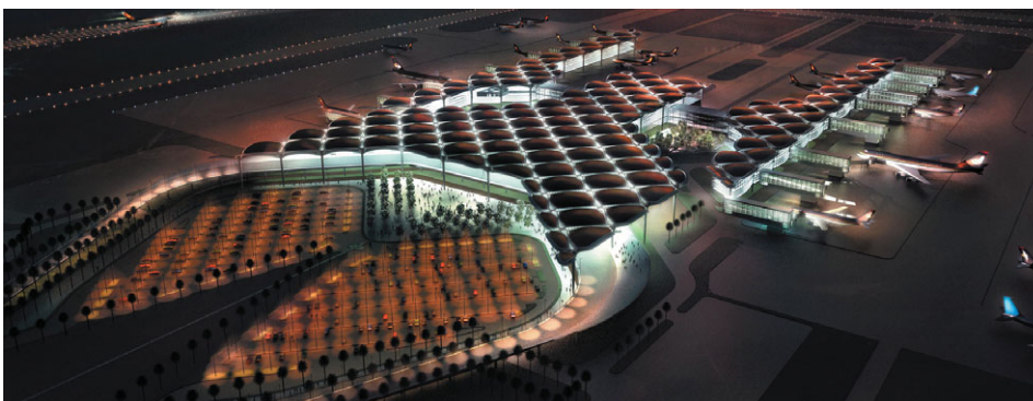
New Doha Airport enjoys ambitious security to match the design of the terminal.
